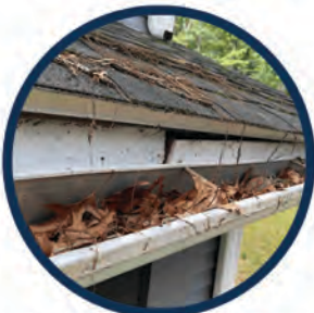
REDUCE ROOF DAMAGE
